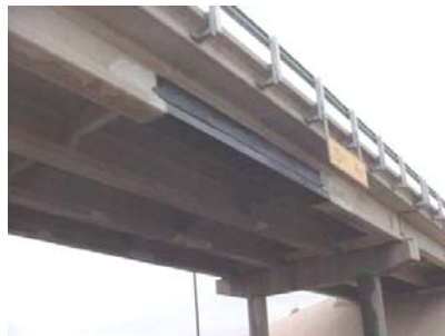
b) A continuous CFRP "U" wrap was used.
