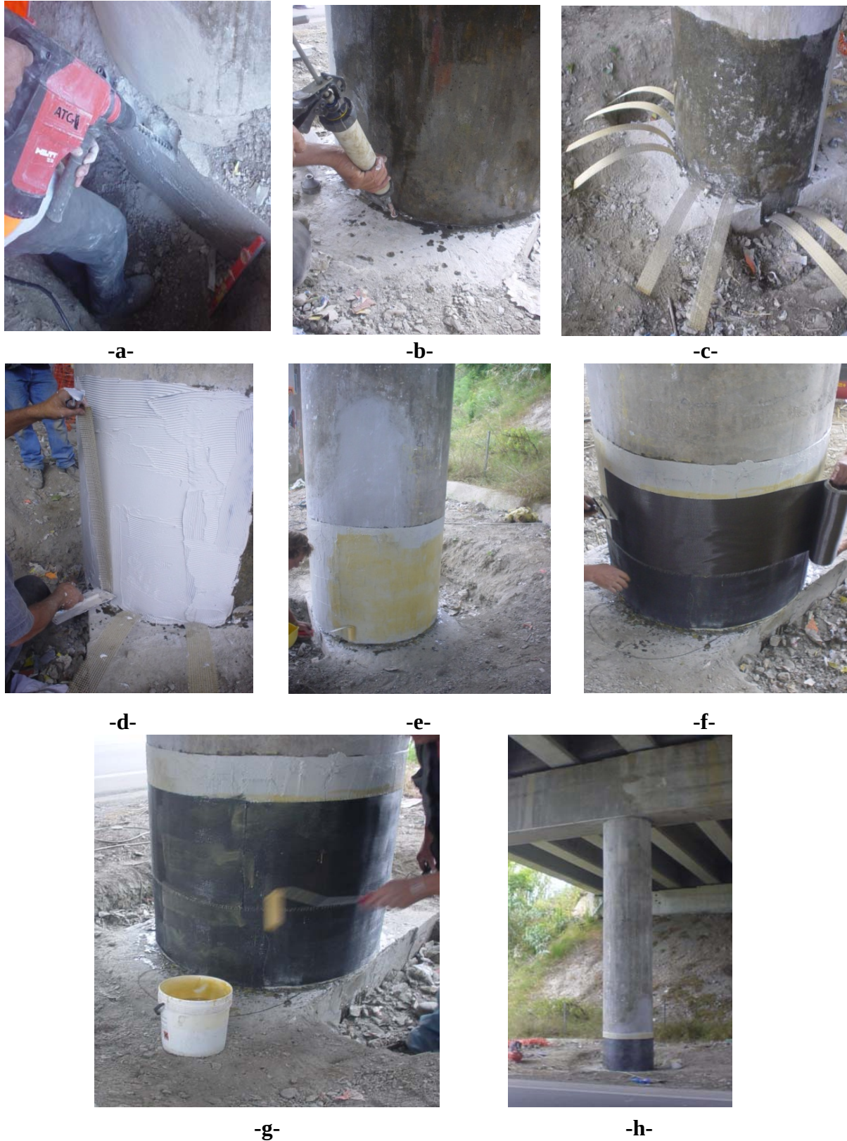
Fig.19 —Innovative materials intervention: application phase
