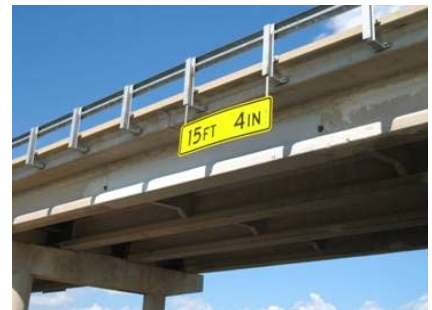
c) The repaired beam after 5 years later.
