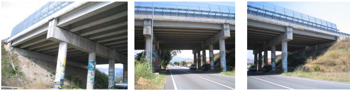
Fig. 1—“Torrente Casale” bridge, on the Salerno-Reggio Calabria Highway
