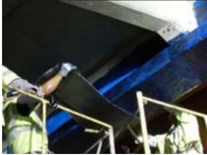
Fig. 1 —Wet layup installations
