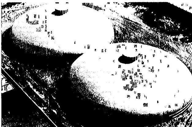
Fig. 1-1—Ellipsoidal shell domes for trickling filters, Hibbing, Minn., 150 ft span (author's photograph)
