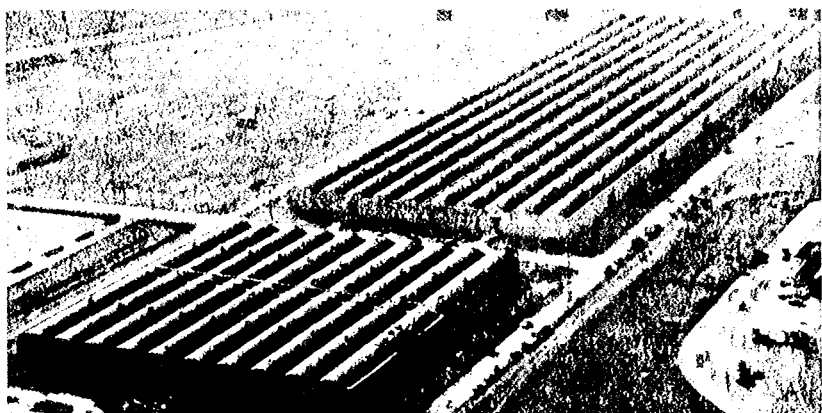
Fig. 1-4—Cast-in-place shells for US Government installation proved competitive with precast concrete structure (author's project)
