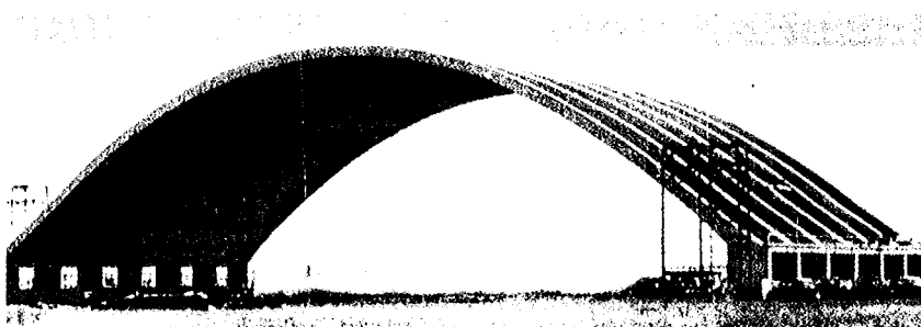
Fig. 1-2—Shell units for aircraft hangar of US Air Force, clear span of 340 ft was longest at that time, stiffening arches restrained by heavy buttresses follow catenary (photographed by author) (similar hangars for American Airlines of 260 ft span, engineered by Ammann and Whitney, followed the same year)
