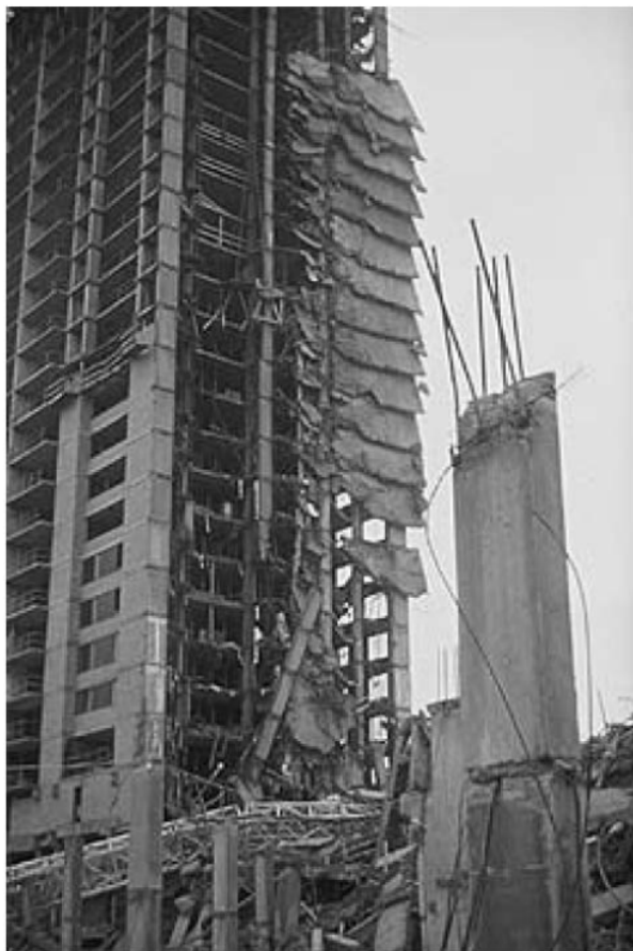
Figure 4 – Skyline Plaza/ Bailey's Crossroads Collapse (photo courtesy Nick Carino of NIST)
