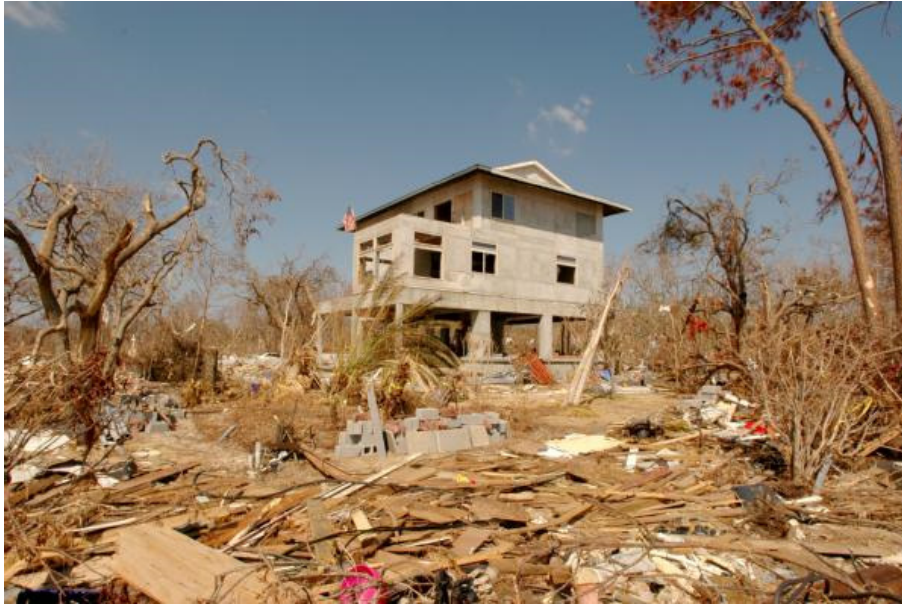
Fig. 3—This concrete house (under construction during hurricane Katrina) was the only house left standing in the neighborhood (photo courtesy of John Fleck, FEMA)
