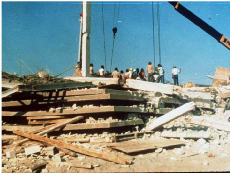
Figure 6 – Harbour Cay Condominium Collapse (photo courtesy Nick Carino of NIST)
