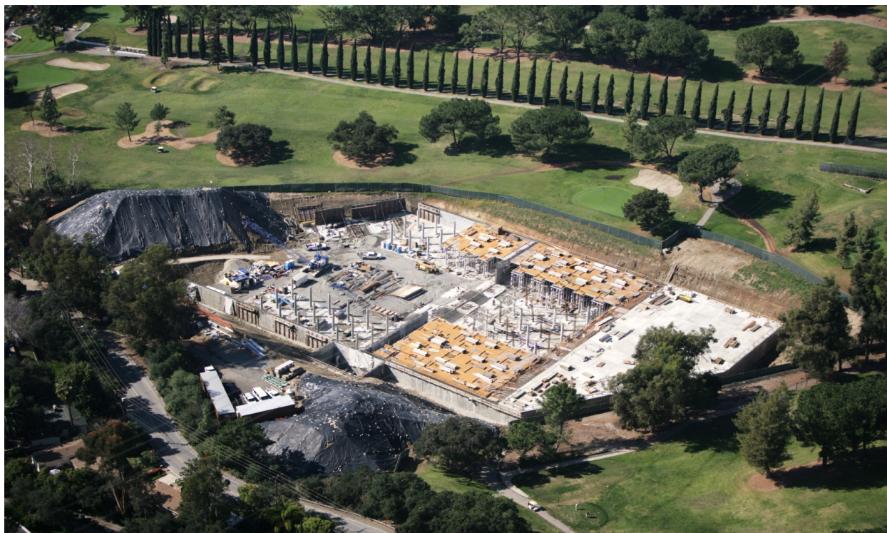
Figure 7-- Aerial photo February 11, 2009
