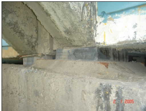
Figure 4 - Replacement of damaged Bearings with new
