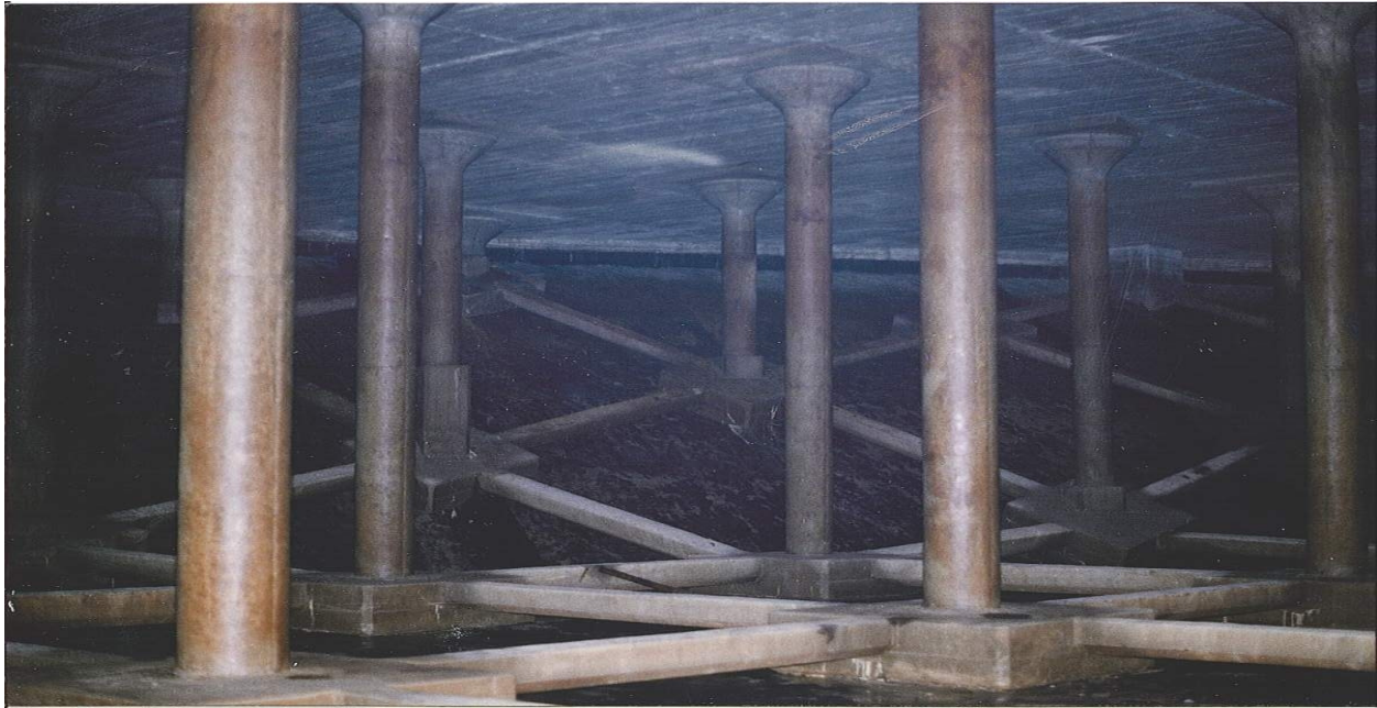
Figure 2-- Interior of existing reservoir
