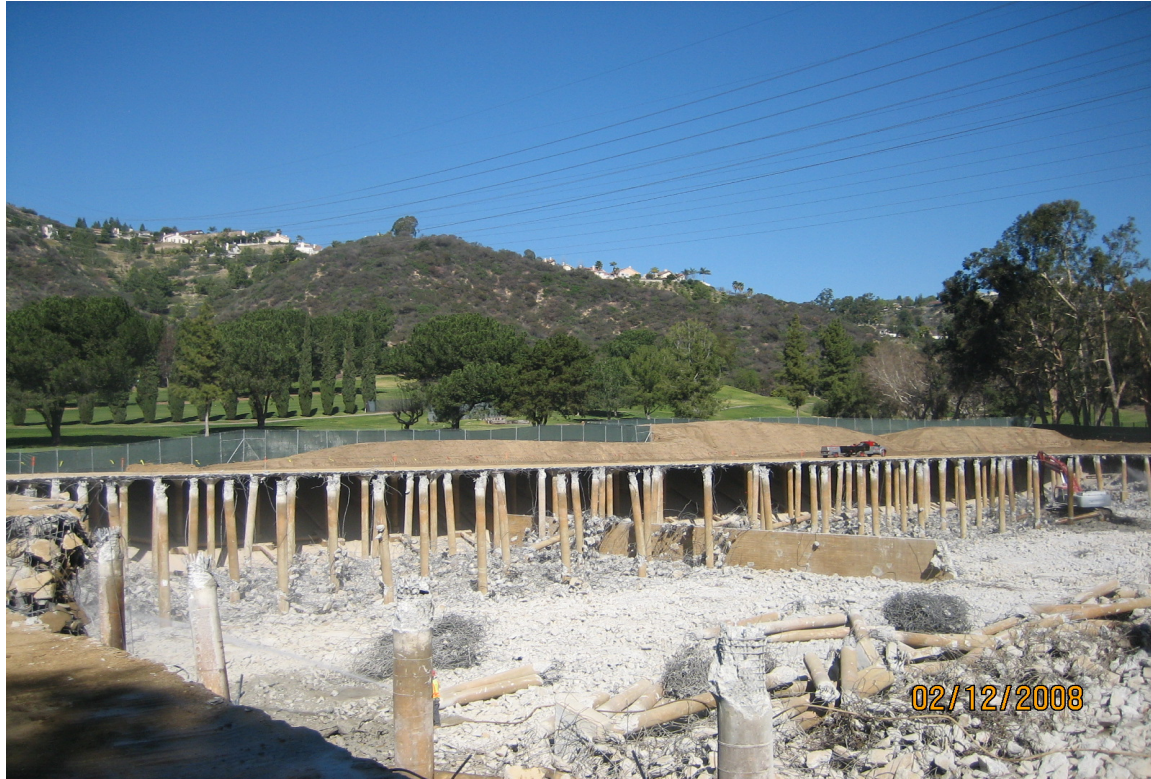
Figure 6-- Steel stockpile for recycling and crushed concrete, half height dividing wall in the middle
