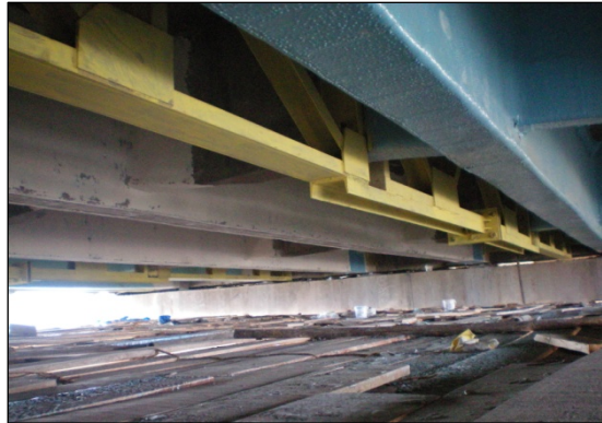
(a) Connection of Truss over Diaphragm Beam
