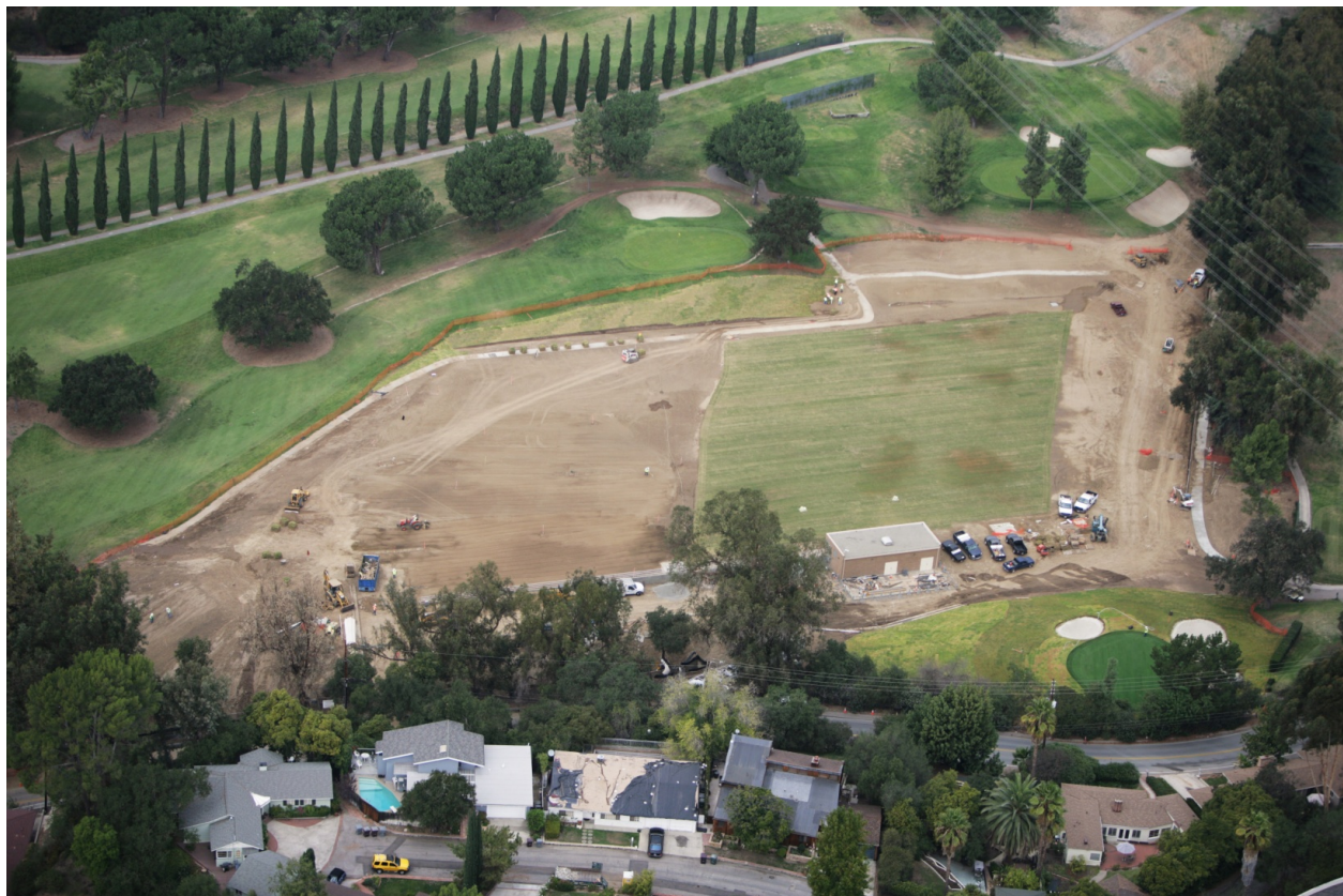
Figure 10-- Aerial photo November 14, 2009, with sod placed on half the reservoir
