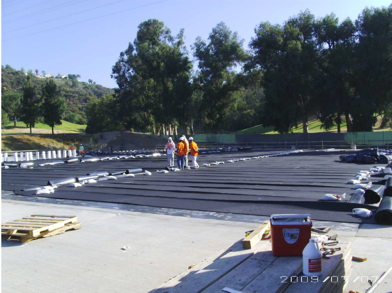
Figure 12-- Application of bituminous sheet membrane on roof prior to earth cover
