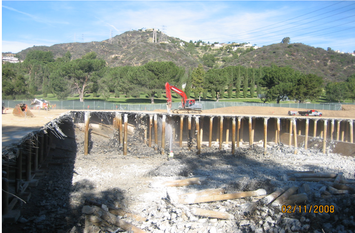
Figure 5-- Demolition of existing reservoir in progress along with dust control mitigation
