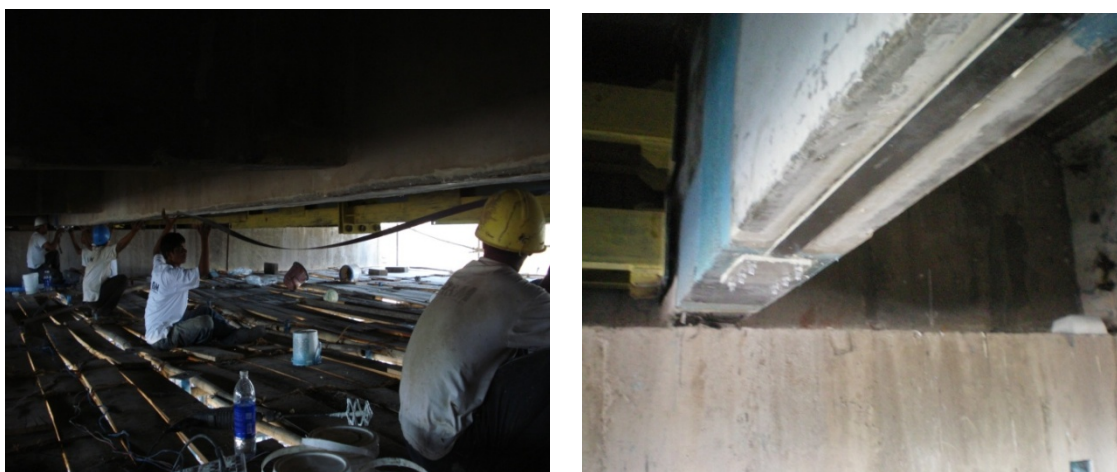
Figure 5. Pre-stressing in process and the finished laminate with anchor plates at end.
