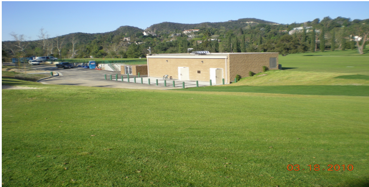
Figure 9-- Pumping station building and access to reservoir
