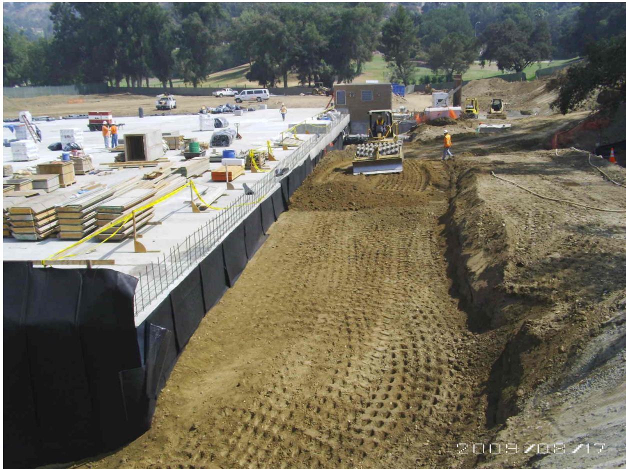
Figure 11-- Backfill in progress against walls with membrane waterproofing
