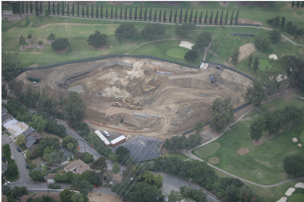
Figure 4-- Excavated site, construction trailers in the foreground, L shape, along with stockpiled material for backfill covered with plastic
