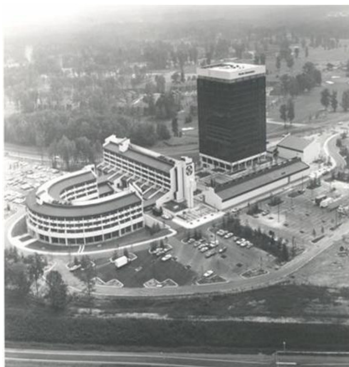
Photo 5- 20-story Office Building- Un-bonded Post-Tensioned Flat Plate (Banded System) and Hotel Building- One-way un-bonded post-tensioned slab, Reston, Virginia 1972
