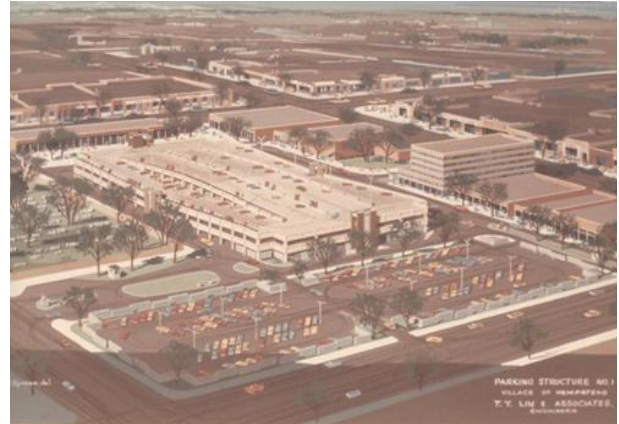
Photo 2 - Parking Structure (Un-bonded PT one-way Slab) Hempstead, Long Island, NY -1968
