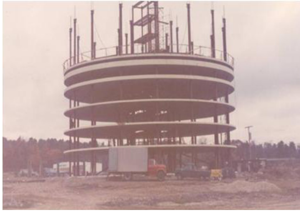
Photo1- Two-way Post-Tensioned Lift-Slab Long Beach, CA – mid 1950's
