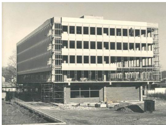
Photo 4- Un-bonded Post-Tensioned (Banded System) Flat Plate Office Building, Danbury, Conn 1971
