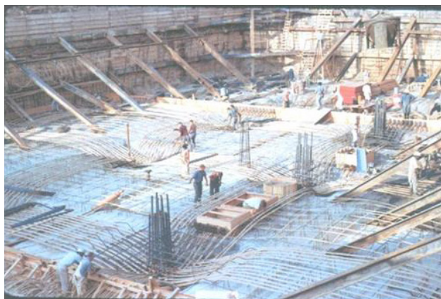
Photo 6- Un-bonded Post-Tensioned Flat Plate Mat Foundation, Washington DC, 1969-70
