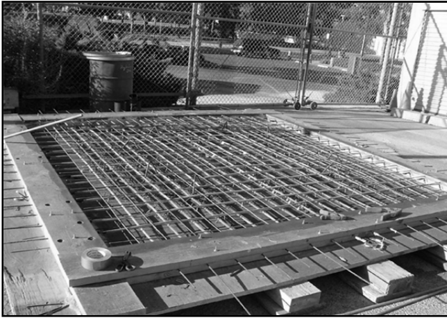
Photo 7- Form- Post-Tensioned-Strands- Reinforcements (at CSUF)
