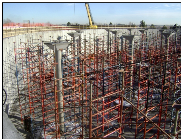
Figure 11—Preparing for the internally cured concrete Contractor used IC even though not specified.
