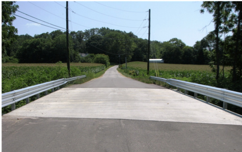
Figure 5—Internall cured bridge deck with no observed cracks after 1 year of service 30
