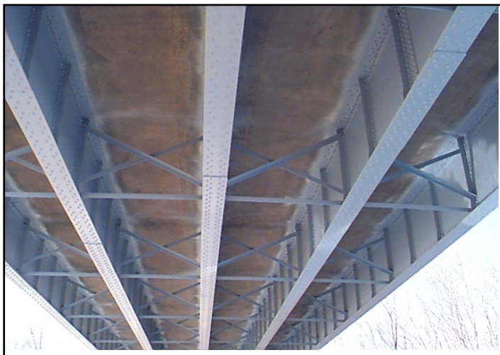
Figure 4—High absorption limestone aggregate bridge concrete. No sign of cracking.
