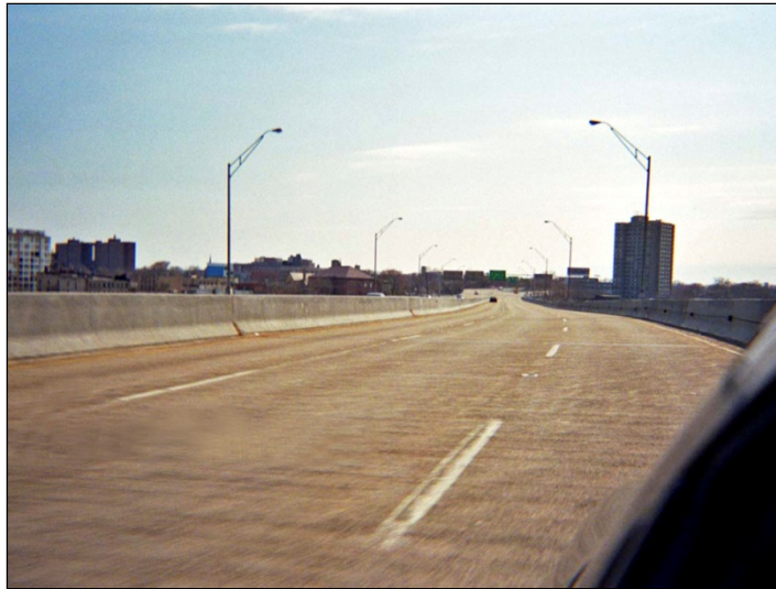
Figure 3—No sign of cracking. Main Avenue Bridge
