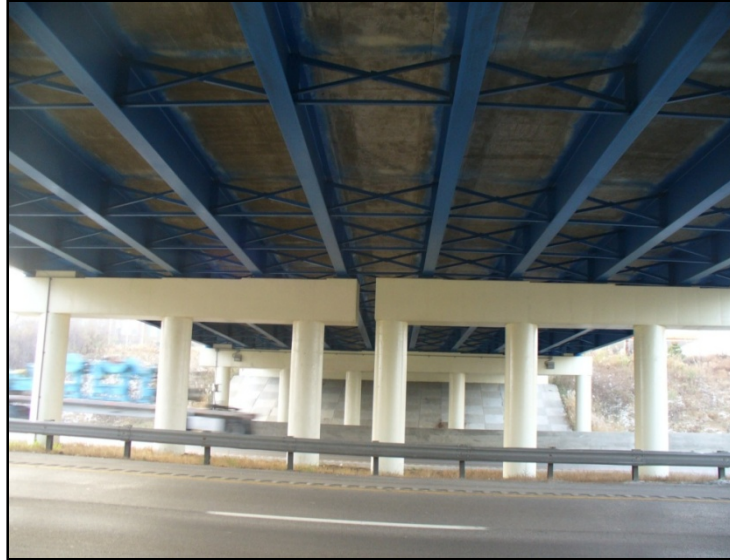
Figure 5—Saturated lightweight fine aggregate internal curing. Compressive strength is 20% greater. No sign of cracking.
