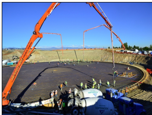
Figure 10—Denver Water Storage Tanks. Internally roof. cured monolithic slab placement
