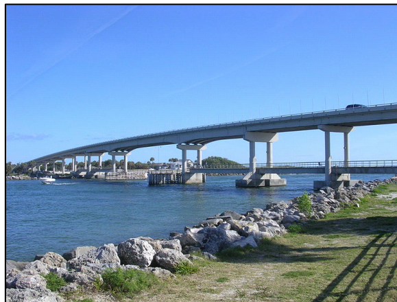
Figure 13—Sebastian Inlet Bridge, FL. Carbonation was less in the lightweight concrete portion of the span.
