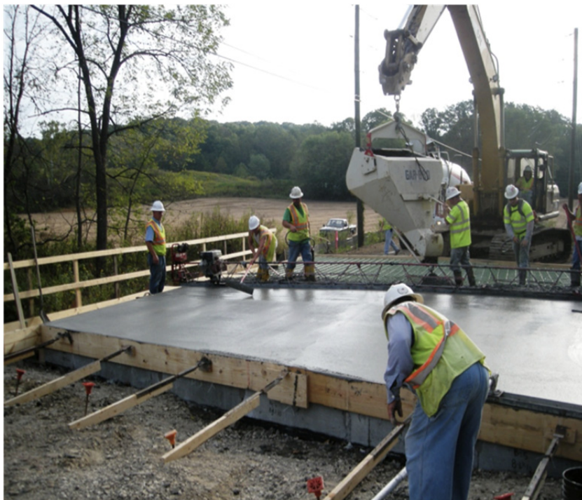
Figure 3—Placement of internally cured bridge deck concrete near Bloomington IN 30
