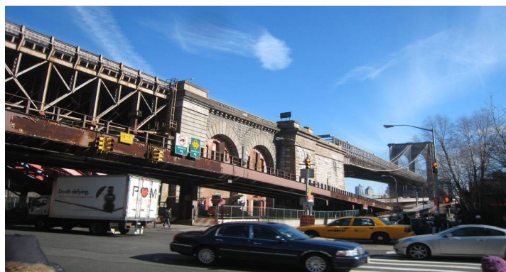
Figure 2 – Masonry arch approach structures on the Manhattan side of the Brooklyn Bridge.
