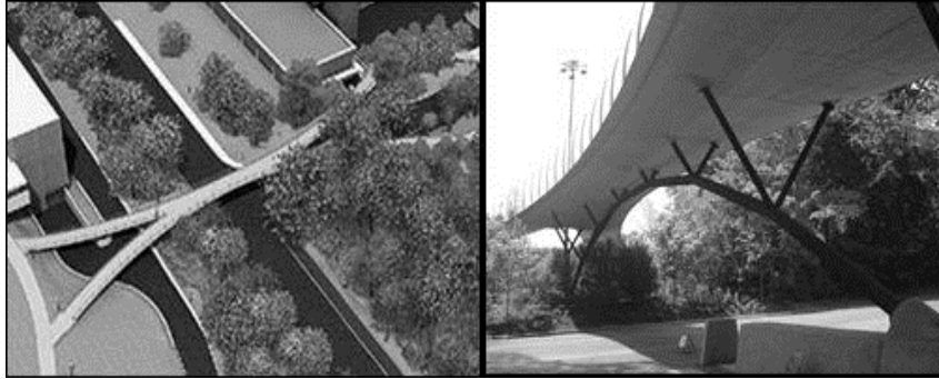
Figure 13–Streicker Bridge. Right: Photograph. Left: Rendering, courtesy of Facilities of Princeton University.
