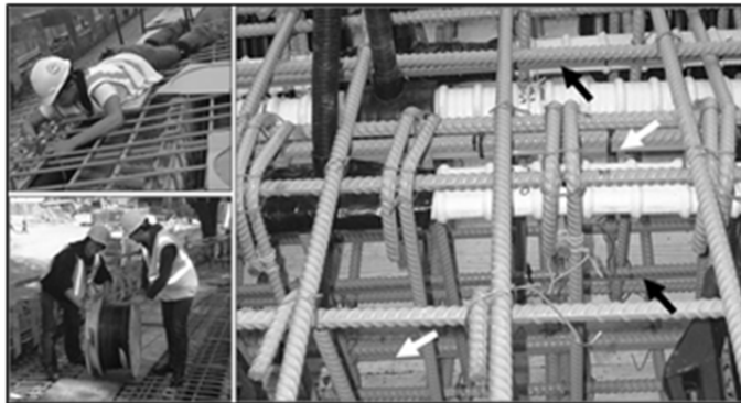
Figure 15—Photographs taken during sensor installation. Top left: Student installing sensor. Bottom left: Students installing extension cable. Right: Parallel discrete and distributed sensors installed on rebar (Glisic et al., 2011).
