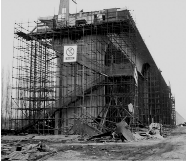
Fig.12 Construction of post-tensioned beams in Datong-Xi'an high speed railway in winter
