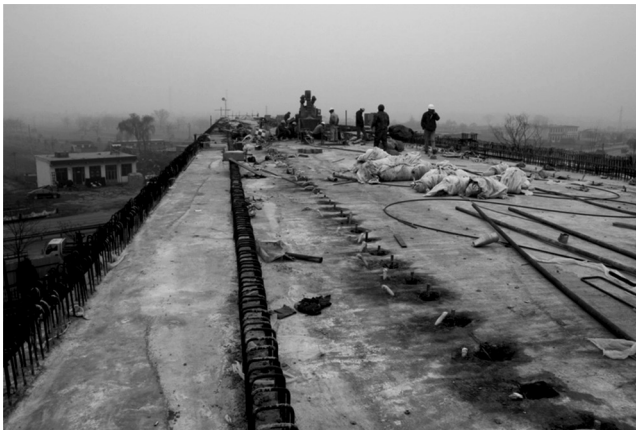
Fig.13 Construction of post-tensioned beams in Datong-Xi'an high speed railway in winter
