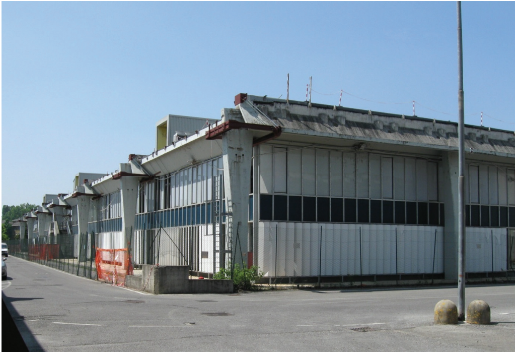
Figure 6 –The part of the Olivetti factory with structural consolidation works
