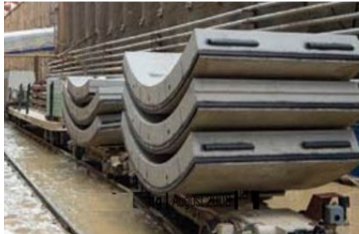
Figure 4: Precast Concrete Segments prior to transportation to Tunnel Boring Machine.
