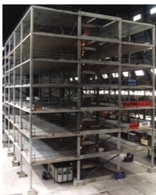
Figure 3: Seven storey reinforced concrete building constructed in Cardington.
