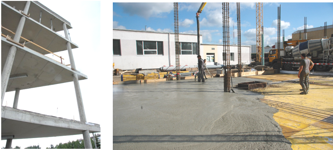
Figure 3: Applications of elevated flat slab using steel fibres as primary reinforcement.
