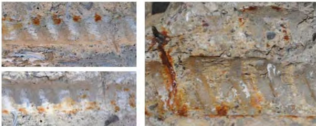
Figure 9 — The interface of the concrete ahead of the steel bar ribs for the CFRP wrapped beam
