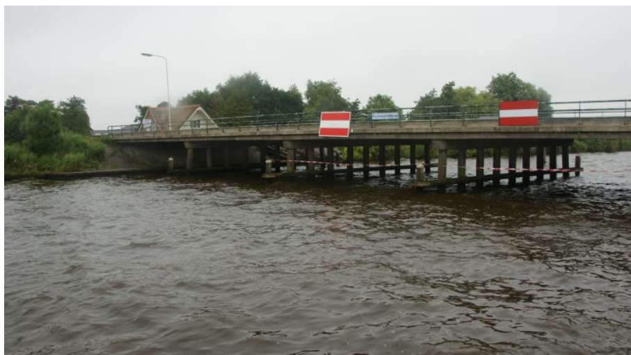
Figure 4 — Ruytenschildt Bridge in 2014.
