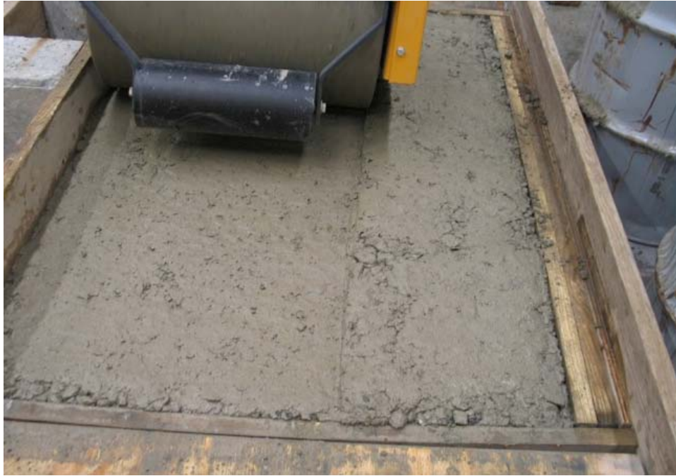
Figure 3 – Compacting RCC lift with single drum vibratory roller
