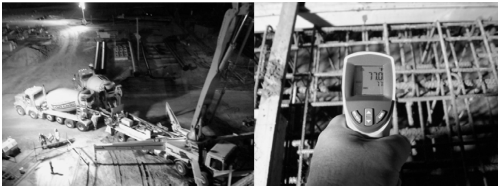
Figure 7 Concrete temperature in the form during nighttime placement.
