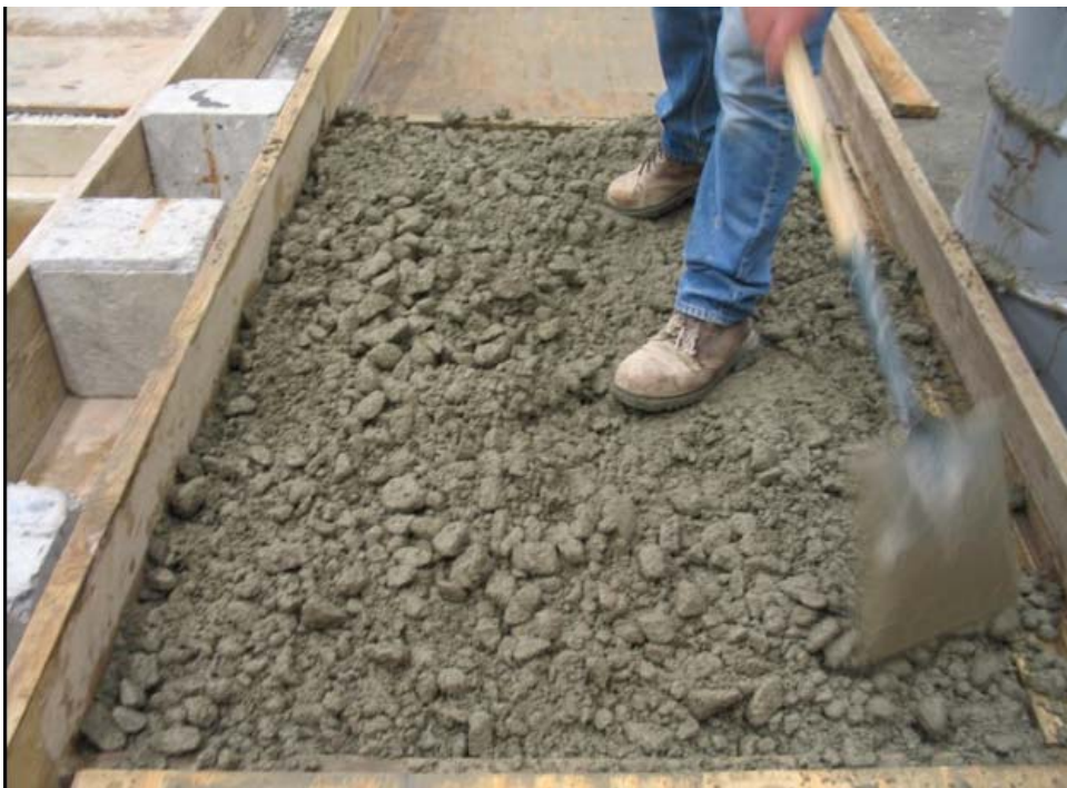
Figure 2 – First lift of RCC placed in test panel form
