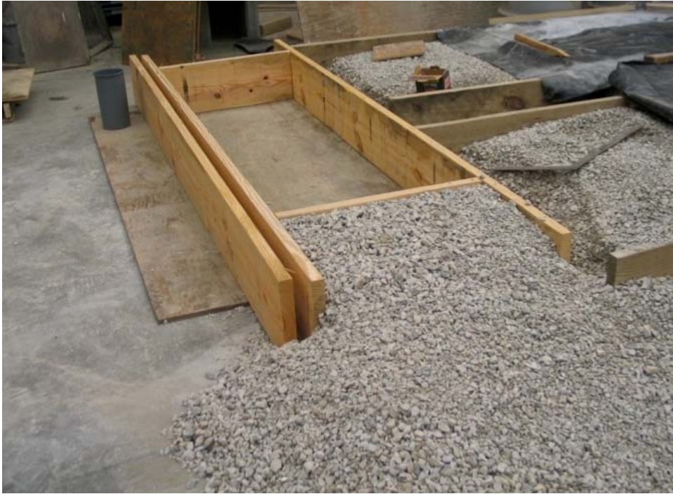
Figure 1 – Forms and bracing for RCC test panel
