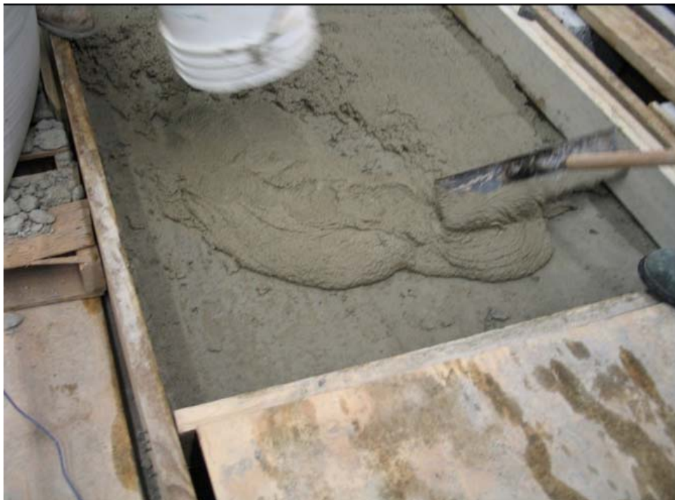
Figure 4 – Applying bedding mortar joint treatment after joint surface has been exposed for required time at designated temperature
