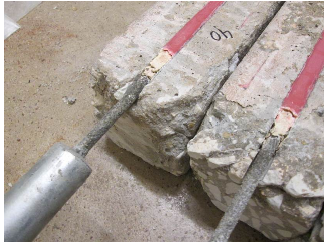
(b) Scaling/spalling at specimen ends
