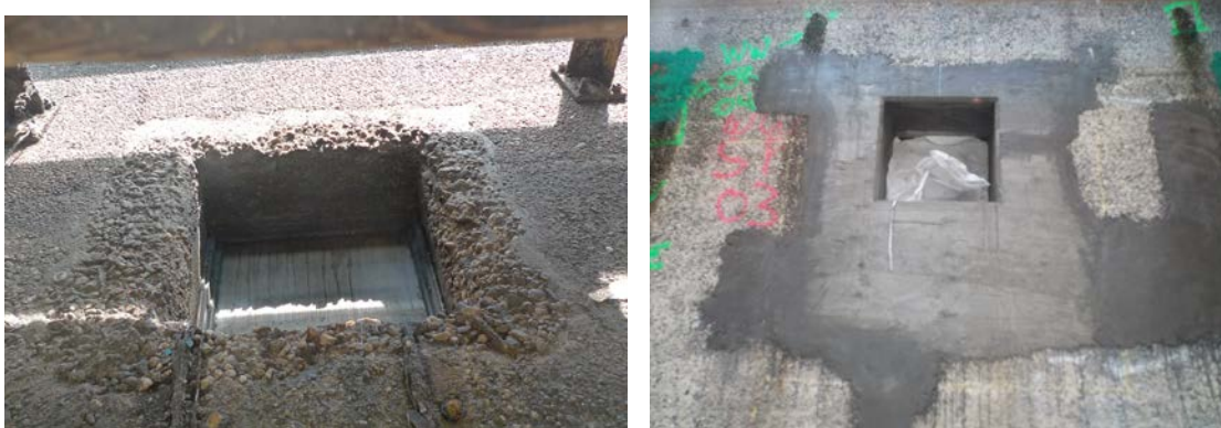
Figure 2 – Exposed corroded reinforcing steel bars and repairs.
