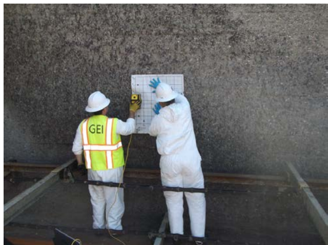
Figure 9 - GPR: Identify internal faults, rebars, hidden piping
