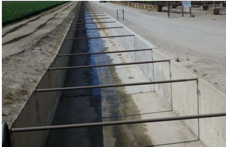
Figure 1- Cantilever wall sections forming a flood control channel.
