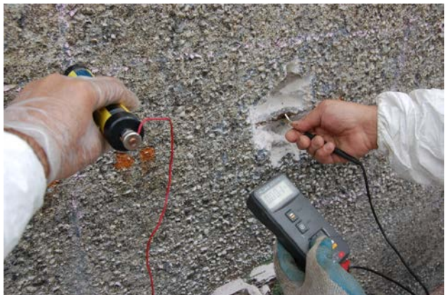
Figure 10 - Half-Cell Testing: Measurement of corrosion potentials
