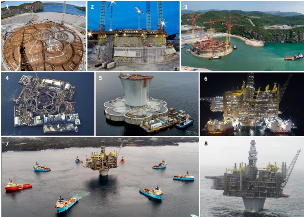
Fig. 8 – Construction phases –Hebron Platform
