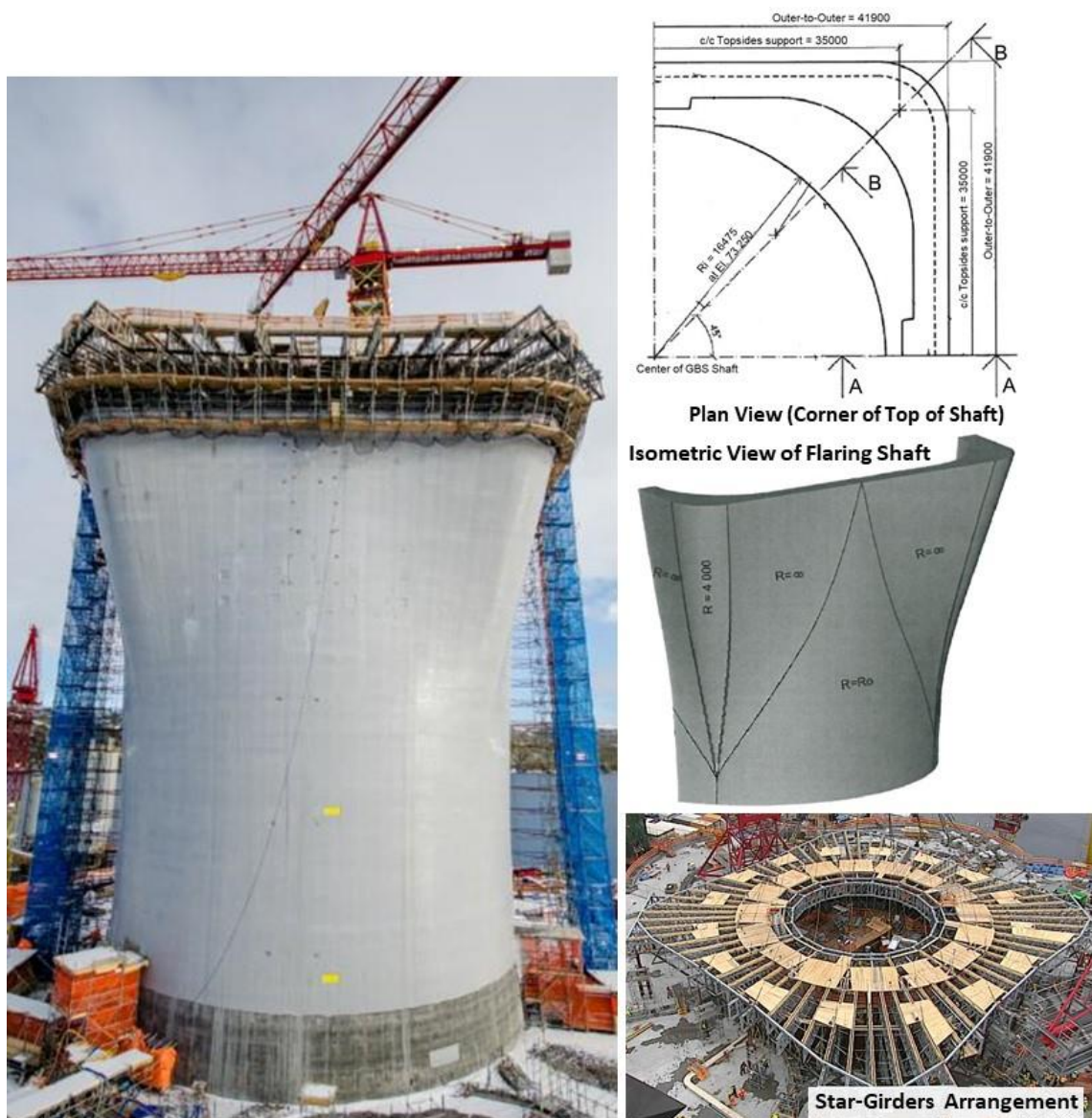
Fig. 7 – GBS shaft unique geometry and star-girder arrangement for shaft slipforming
