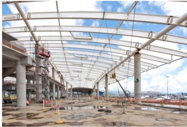
Figure 8 — Site photo of the roof structural steel construction in Zone 2B
