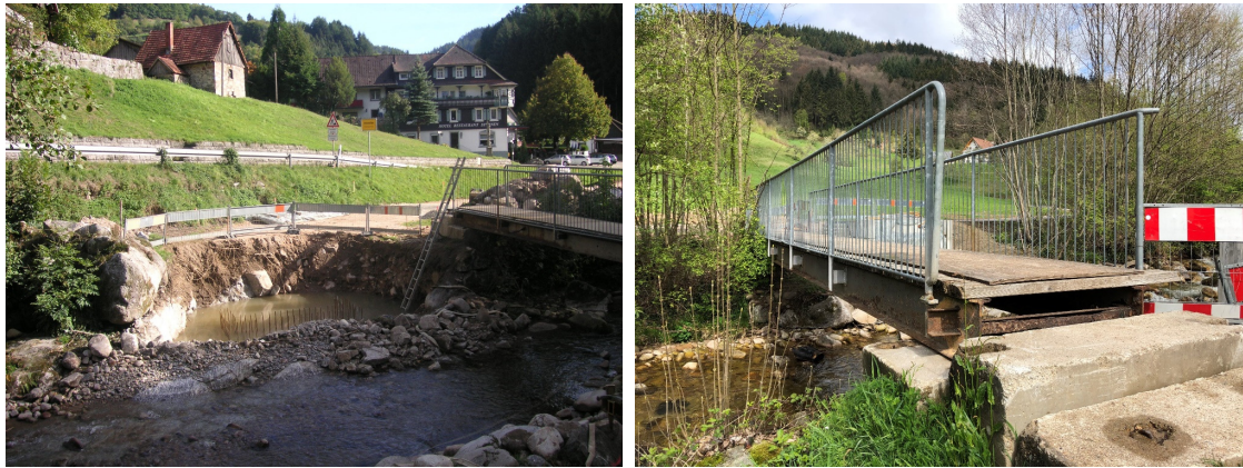
Figure 5 —Site view prior to construction of new bridge; left: construction pit for new foundation (photo: RS Ingenieure GmbH & Co. KG); right: temporary pedestrian bridge (photo: Sergej Rempel)
