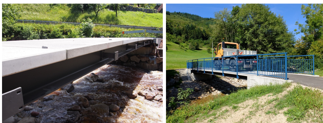
Figure 10 —Site view after installation of TRC deck panels prior to fastening of steel handrail (left, photo: Jan Bielak) and with service vehicle after inauguration (right, photo: RS Ingenieure GmbH & Co. KG)
