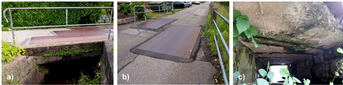
Figure 11 —Situation prior to bridge replacement in Gaggenau, Germany: a) Siedlungsstrasse; b) and c) Heilweg (photos: Jan Bielak)
