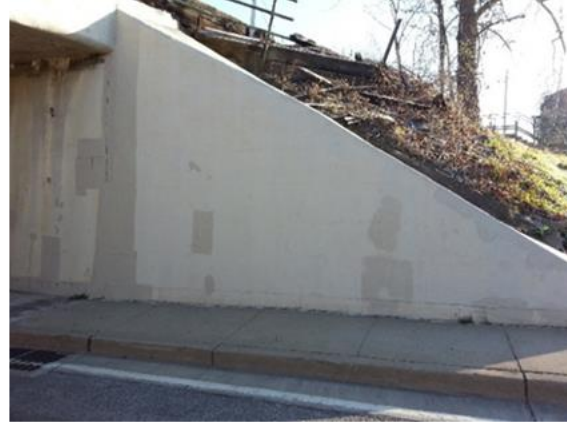
(b) GFRP wrapping on a wing wall
