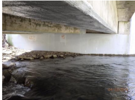
(b) CFRP wraps in underside of a T-beam and abutment #1
