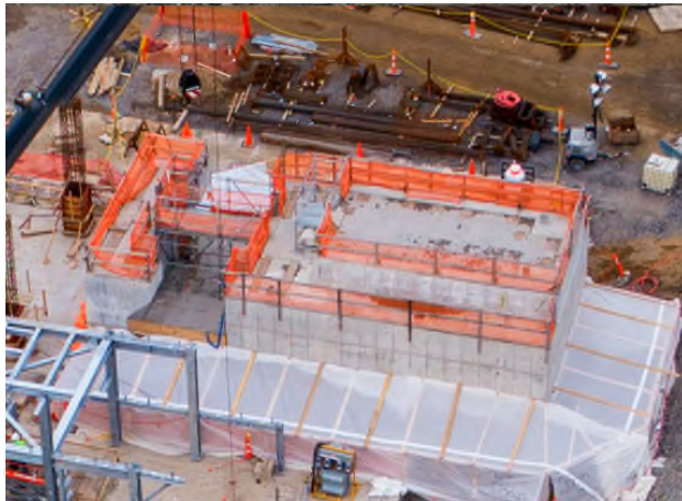
(c) Preparation for constructing the bracket
