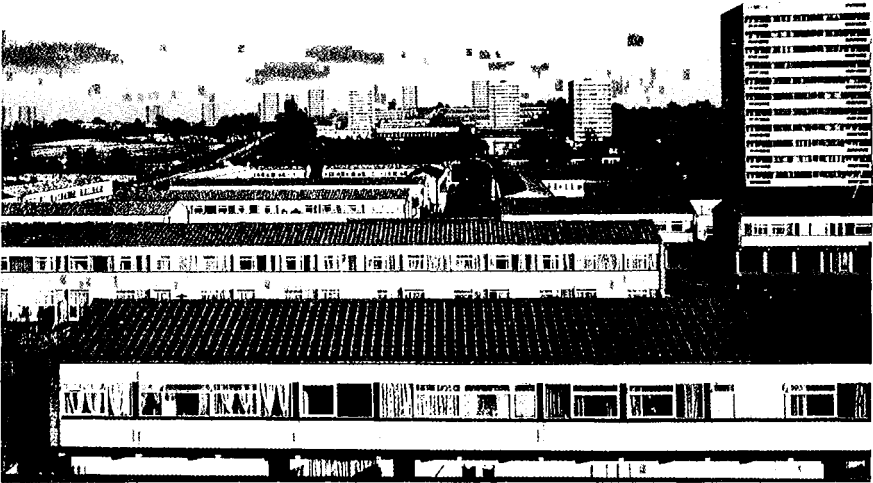
Wall Frame Flats, Birmingham 1964/65. Standard blocks adequately spaced to blend with the surroundings
