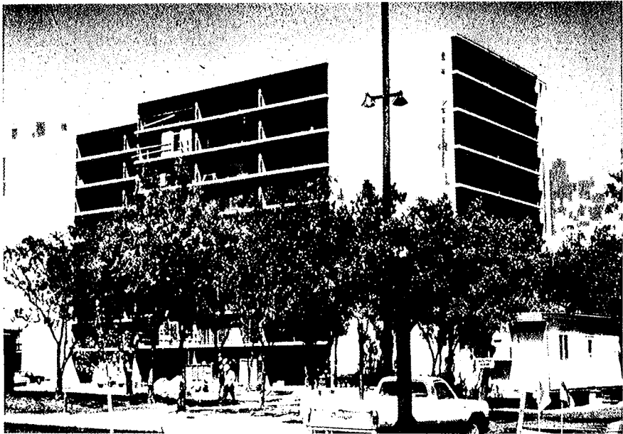
F.C.E.--Dillon System, Sacramento, Calif., HUD Operation Breakthrough, 9 story highrise
