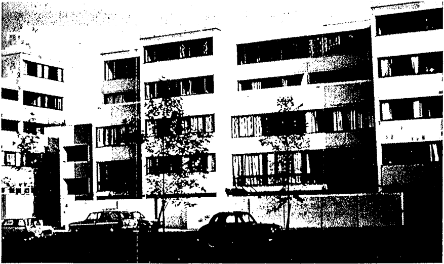
Rouse-Wates System, St. Louis, Mo., Medium rise building for HUD Operation Breakthrough
