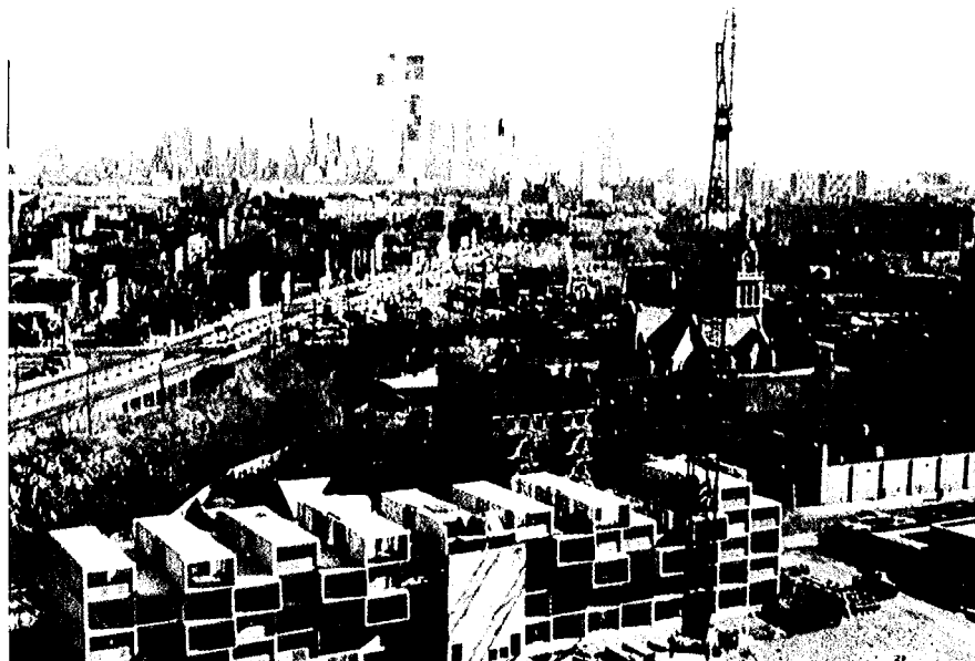
Shelley System, Jersey City, N. J., HUD Operation Breakthrough, 18 story highrise under construction
