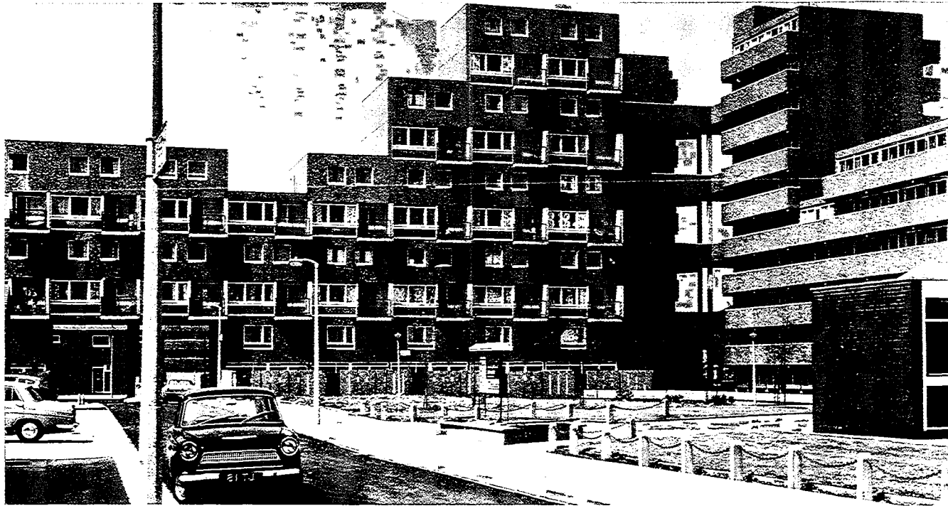
An unwieldy attempt to get character into a lowrise deck access development. Access decks junctions are clearly visible in right center of the picture, built in 1971
