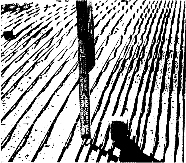
Fig. 3--Screed wires
