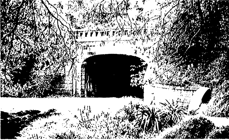
Fig. 5—The Alvord Bridge, designed and built by Ernest L. Ransome in San Francisco, Calif. in 1889, was the first reinforced concrete bridge in the United States. It has been designated an ASCE Landmark Structure. (Photo by Howard Newlon, Jr.)
