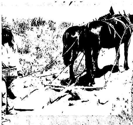
Fig. 9 — Construction methods used on Roosevelt Dam illustrates the notable engineering achievement of these early dams
