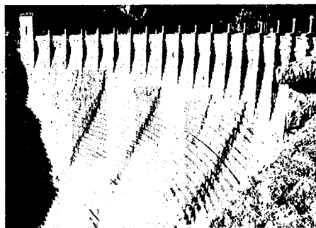
Fig. 6 — Downstream face of Roosevelt Dam built of cyclopean rubble masonry faced with rough ashlar blocks
