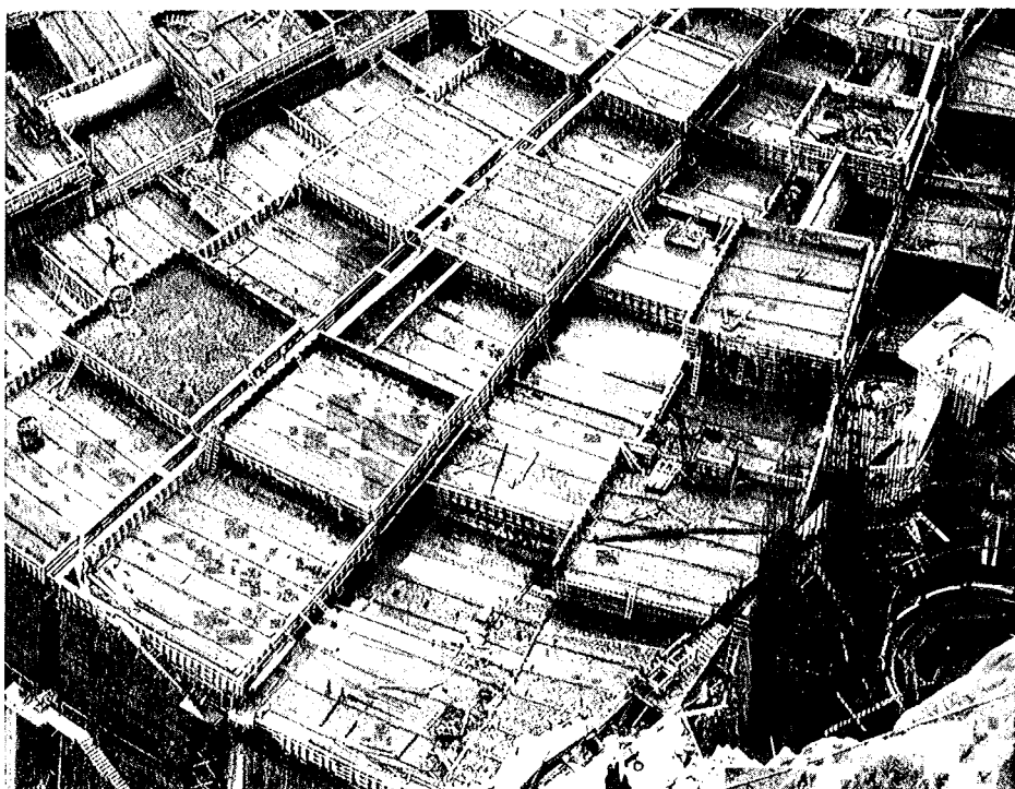
Fig. 14 — Hoover Dam was constructed of columnar blocks with horizontal section as large as 50 x 60 ft
