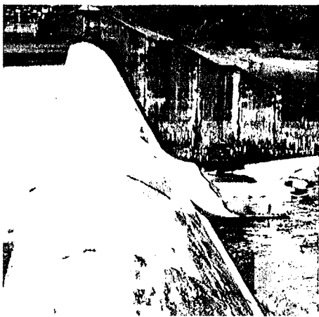
Fig. 4 — Spillway crest and south abutment wall of Hinckley Dam (1948)
