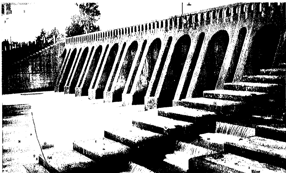
Fig. 16 — Downstream face of Pine River Dam (1928)
