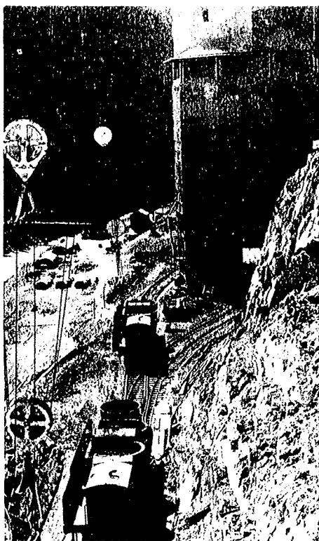
Fig. 16—Concrete cars on trackway along bucket loading dock at Hungry Horse Dam
