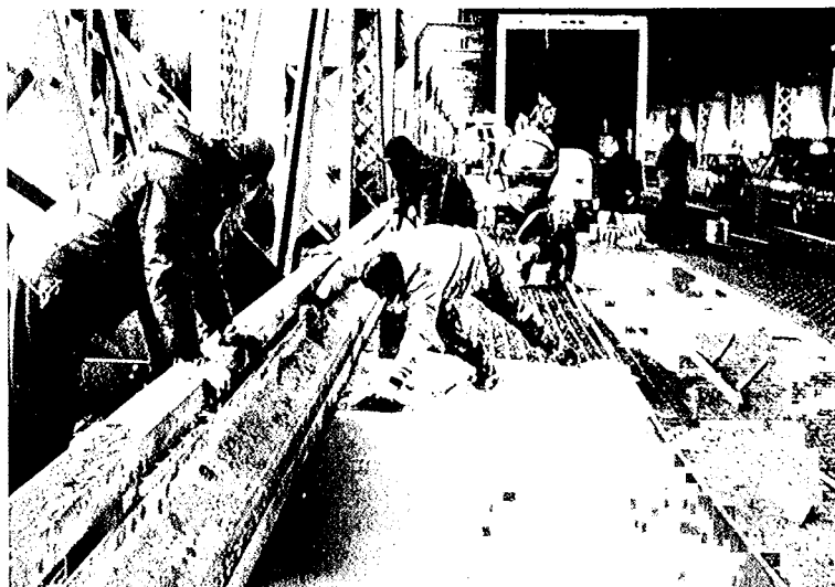
Fig. 19--Application of premixed methyl methacrylate PC overlay on concrete-filled steel grid deck, Queensboro Bridge (59th Street Bridge between Queens and Manhattan), New York City
