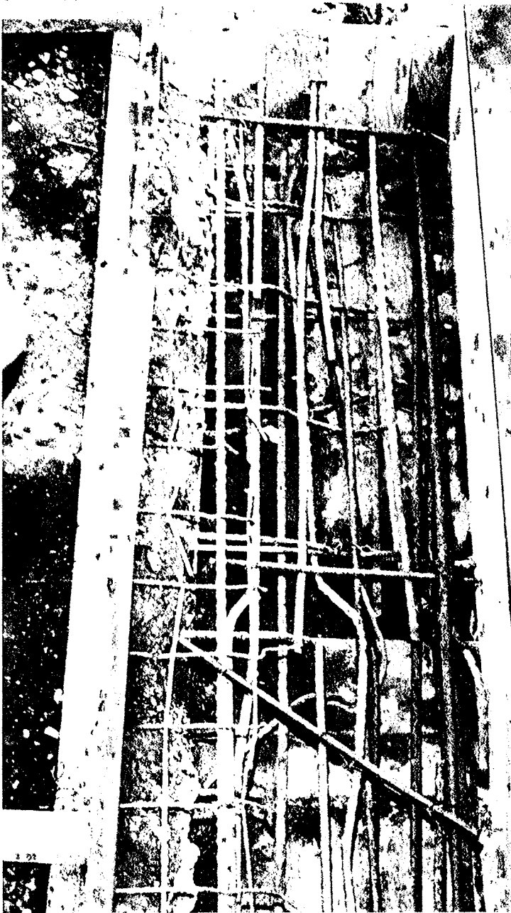
Fig. 1--Full depth hole in bridge deck prior to filling with polymer concrete
