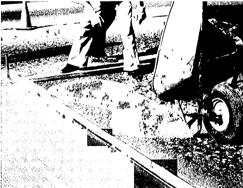
Fig. 18--Application of premixed PC overlay near Donna Pass, California
