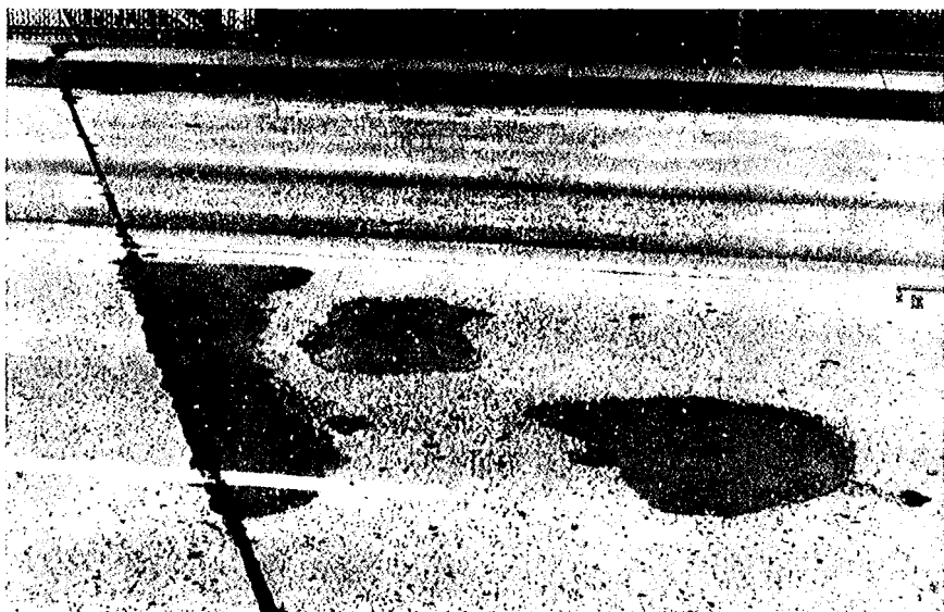
Fig. 9--PC repairs after four years service
