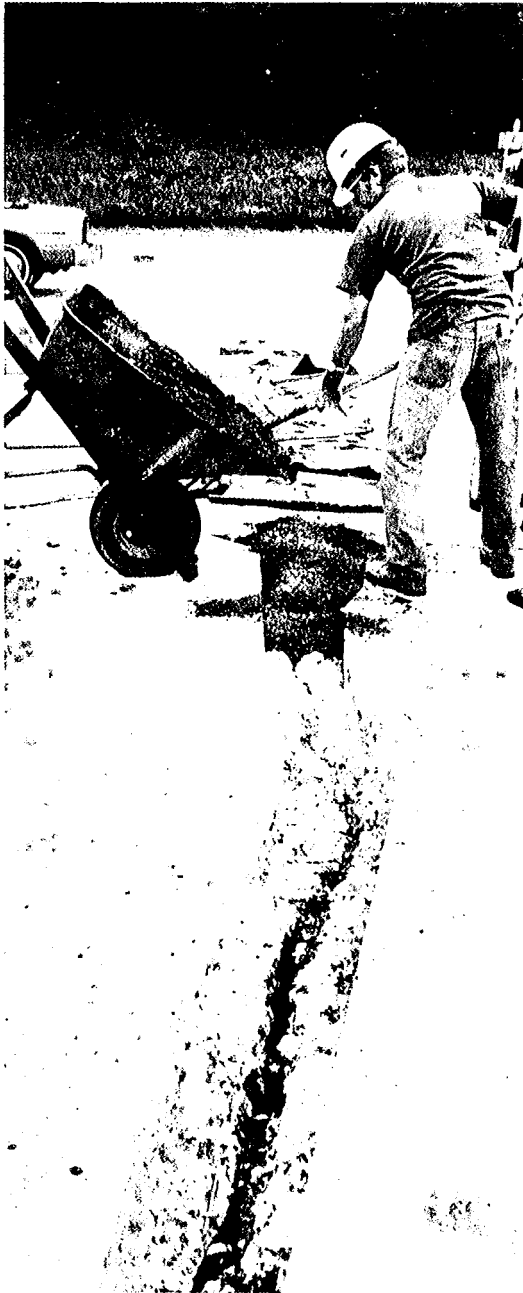
Fig. 12--Repair of pavement cracks with PC
