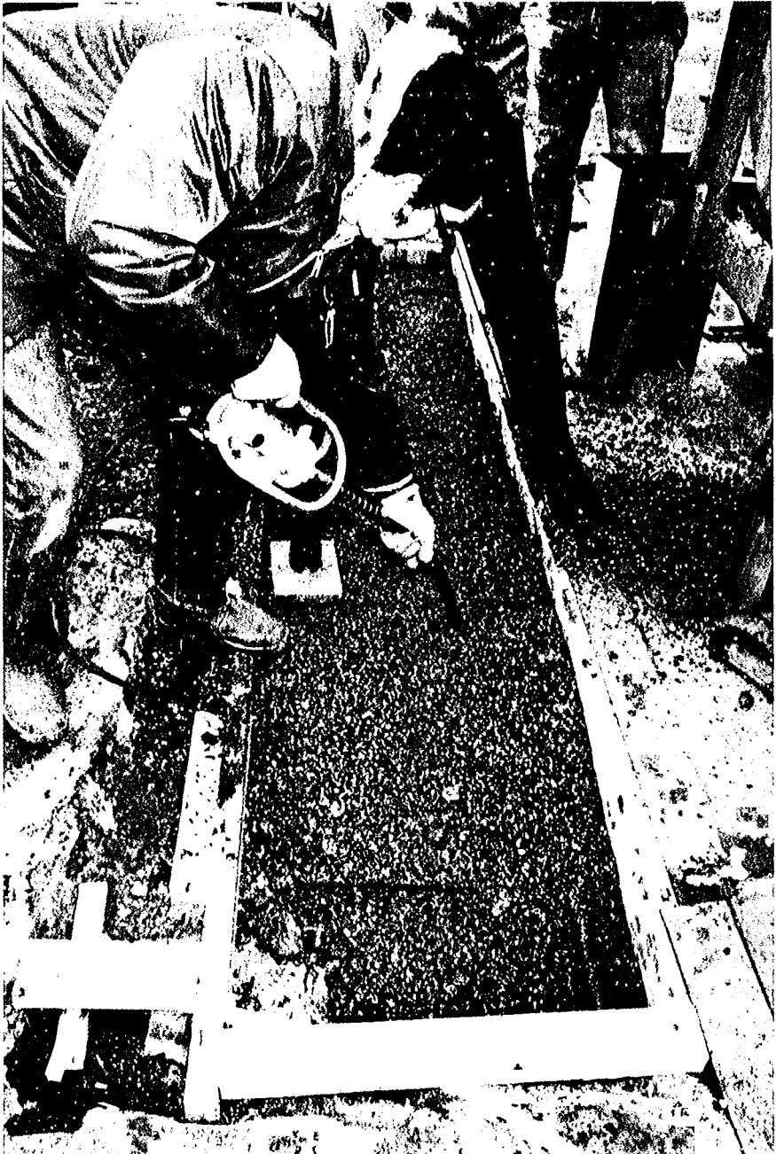
Fig. 4--Compaction of PC using finger vibrator
