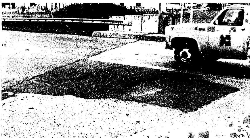
Fig. 10--PC repair after four years service
