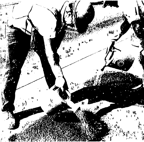
Fig. 7--Monomer saturation of dry aggregate for PC repair by dry pack method
