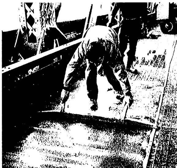
Fig. 19--Application of premixed methyl methacrylate PC overlay on concrete-filled steel grid deck, Queensboro Bridge (59th Street Bridge between Queens and Manhattan), New York City
