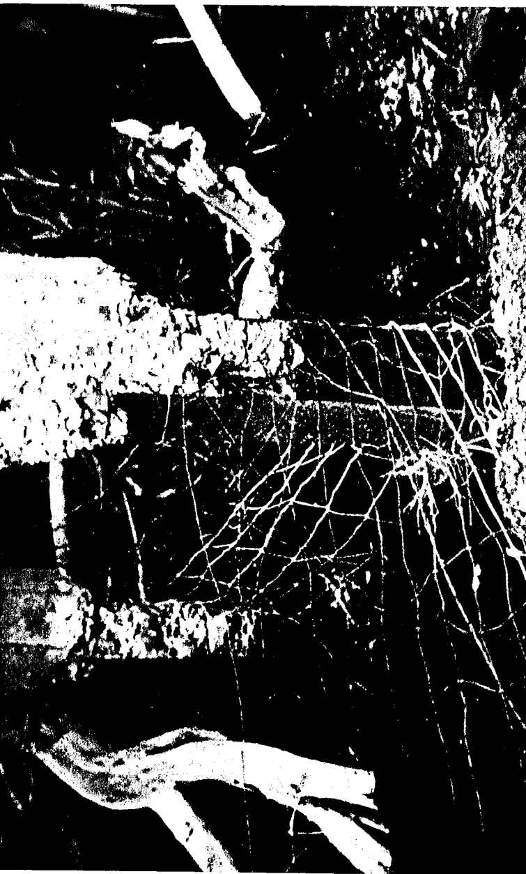
Fig. 1--Sulfate attack on bridge columns. White Wood Creek, Belle Fourche Project, South Dakota
