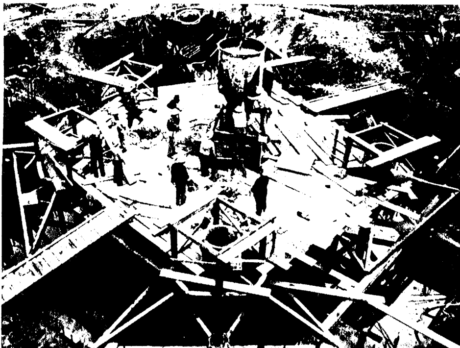
Fig. 2—Placing of the seal and structural floors for a nuclear reactor
