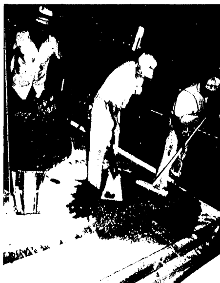
Fig. 15--Filling joints with polymer concrete
