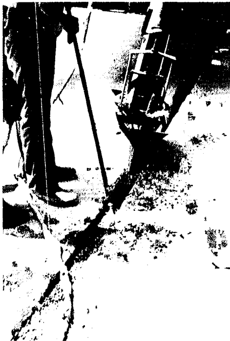
Fig. 8--Placing polymer concrete in trench cut lane joint separation
