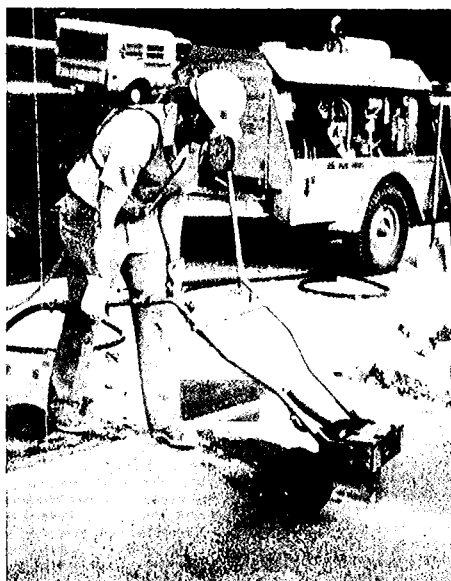
Fig. 16--Preparing longitudinal cracks for repair
