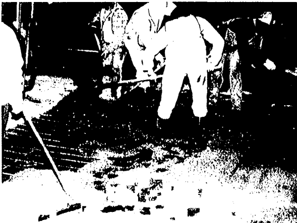
Fig. 10--Placing polymer concrete in full-depth repairs
