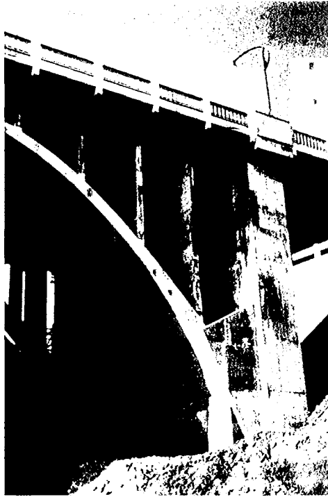
Fig. 5—Completed structure showing part of the repairs and strengthening (1959)
