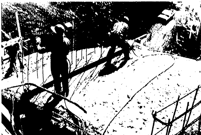
Fig. 3—Preparatory work on the 19-day-old concrete arch (1959)
