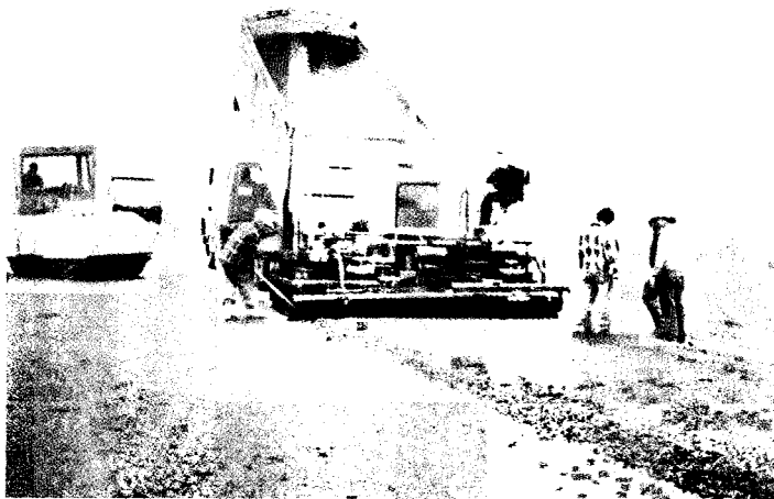
Photo 4—Paving 100 mm of bituminous treated permeable base (O.G.D.L.)
