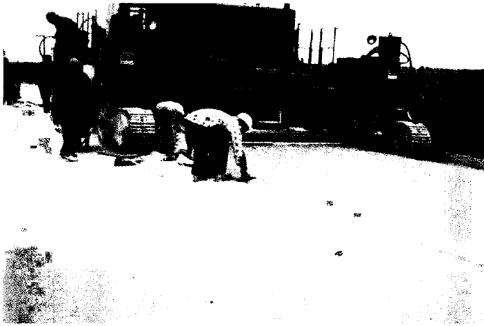
Photo 3—Slipforming E.B.L. and shoulder (sections III & IV)
