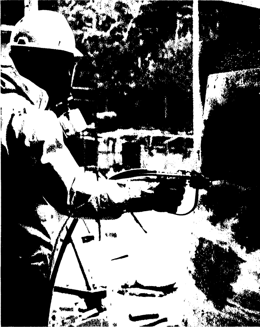
Fig. 5--Safety equipment to be worn by operator during spray application
