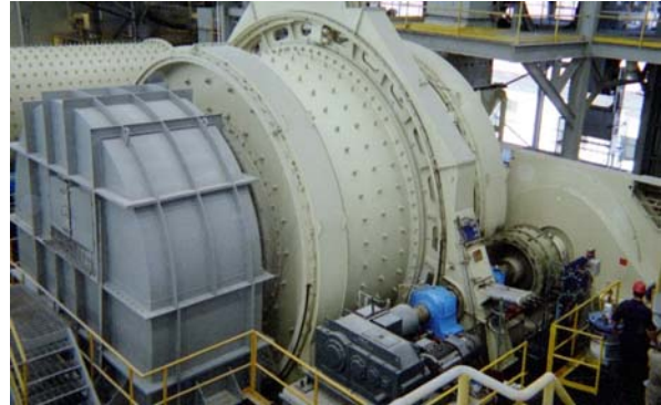
Figure 1. Grinding Mill Installation
