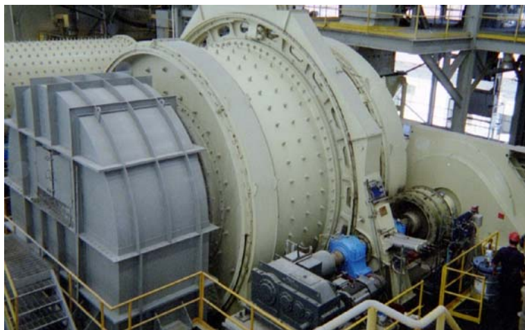
Figure 1. Grinding mill installation
