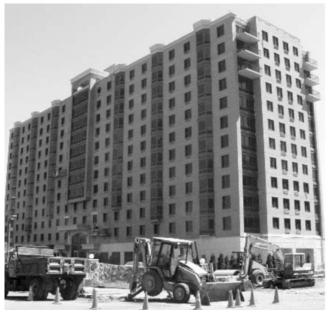
Fig. 1.3 Staggered truss apartment building.
