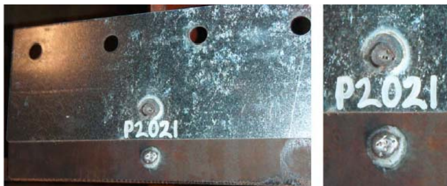
Figure 1.3: Shear weld failure (Guenfoud, 2010).
