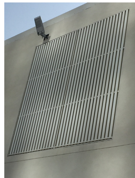
Figure 2. Sand louver with inclined plate, usually called a drain sill. Image courtesy of Ruskin Titus Gulf.
