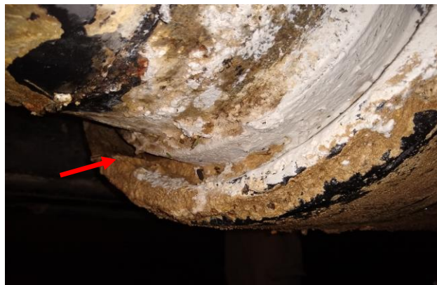
Photograph No. 4 – Location #1, Spot Rust on Pipe Cable
