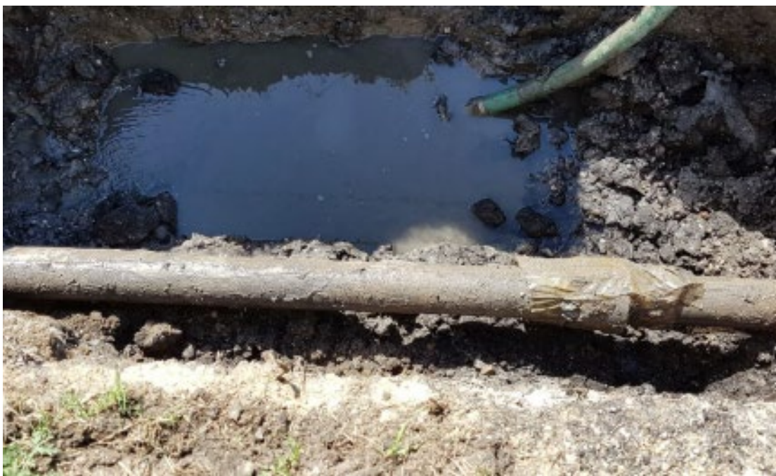
Figure 2: The exposed pipe prior to removal of the polyethylene film. Regular pumping controlled the inflow of groundwater from the surrounding soils.
