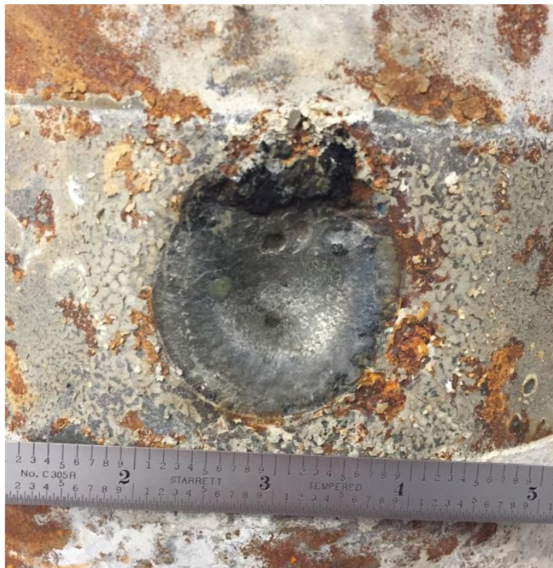
Figure 2: Through wall anomaly
