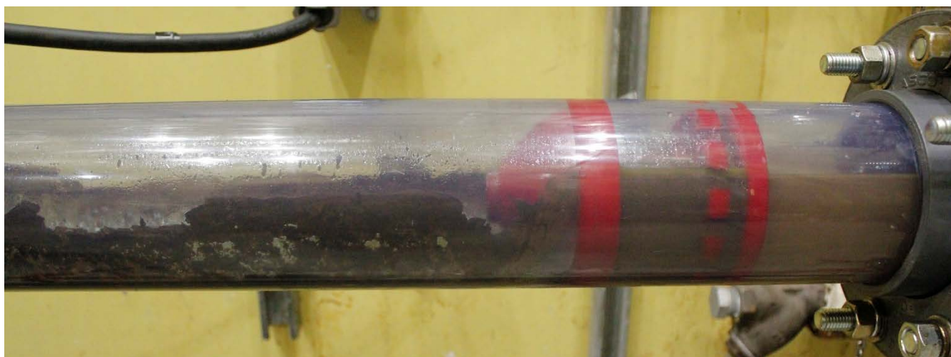
Figure 5: Image of filming pig inside clear PVC pipe section during the commissioning phase of the project with sludge debris in front of the pig (travel from right to left).
