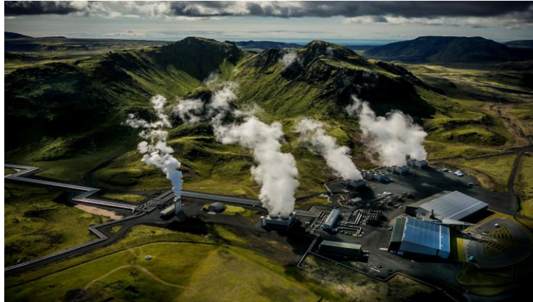
Figure 1: Hellisheidi Geothermal Power Plant Site [13].
