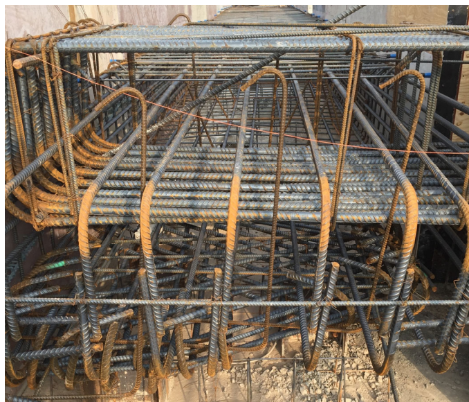
Figure 3: Grade beam to footing construction
