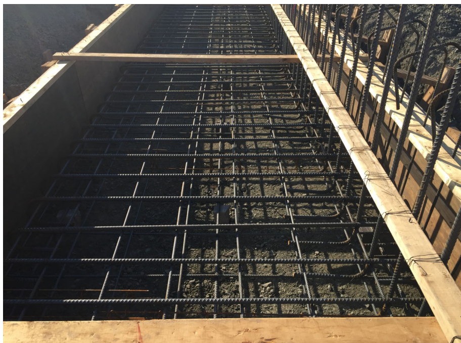
Figure 1: Retaining wall footing
