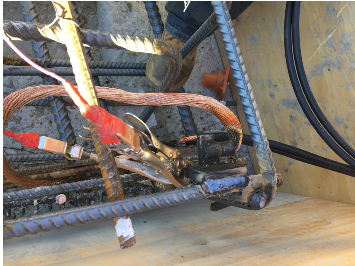
Figure 2: Bonded rebar footing corner
