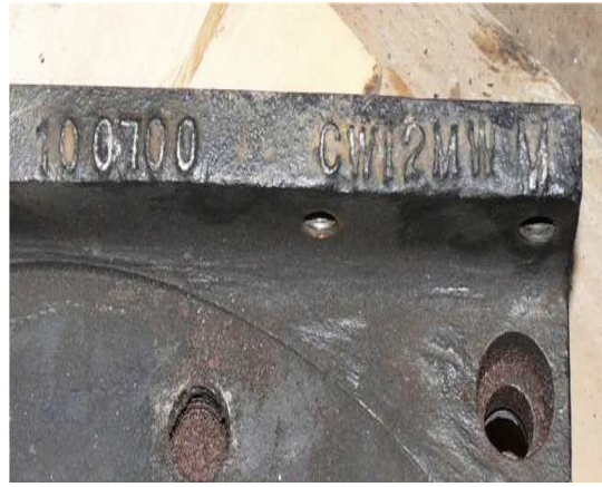
Figure 3: ASTM Casting Grade on valve body
