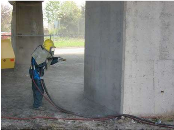
Figure 1: Abrasive Blast Surface Preparation
