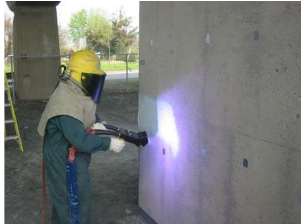
Figure 2: Arc Spray Zinc Anode Installation
