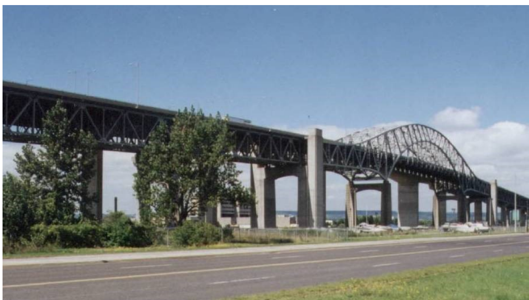
Figure 1: Burlington skyway, Burlington, Ontario, Canada
