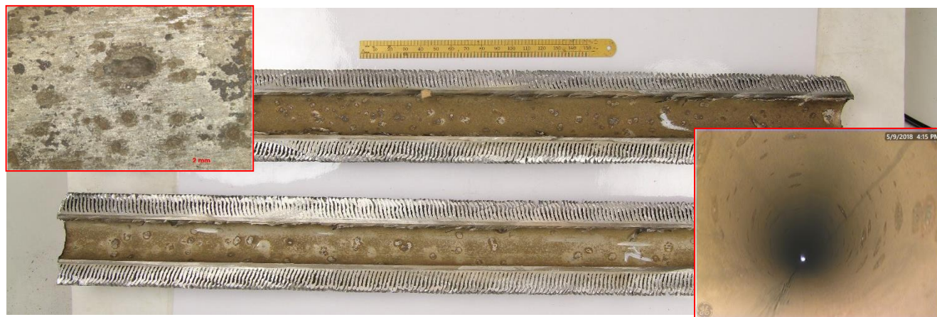
Figure 3: Visual observation of pitting and localized corrosion across the tubes
