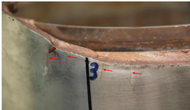
Figure 4: Photograph showing the secondary longitudinal cracks on the OD (arrows).
