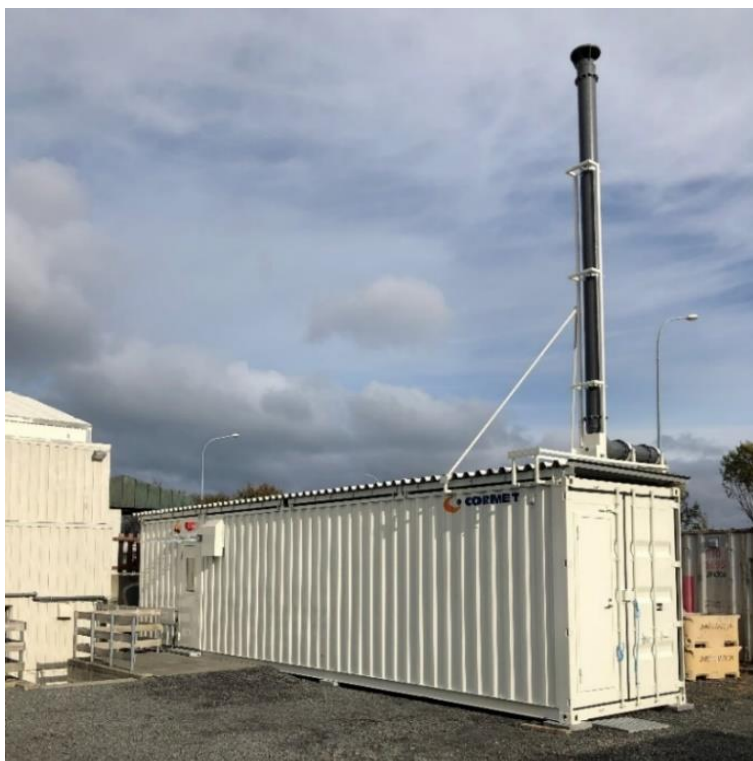
Figure 1: The corrosion laboratory constructed in a 40-foot high-cube container by Cormet Oy, Finland, shipped to Iceland, and installed at the campus of the University of Iceland.
