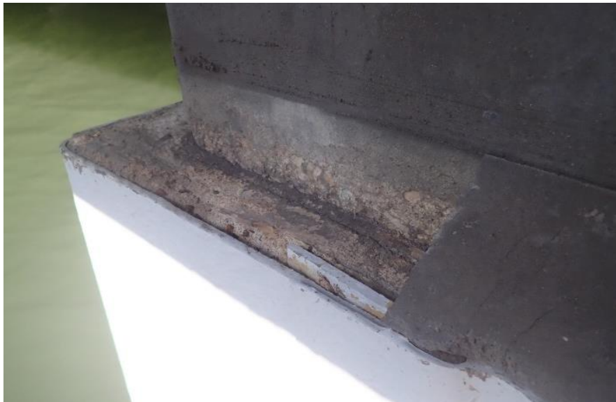
Figure 3: Sloped grout topping removed by hammer sounding
