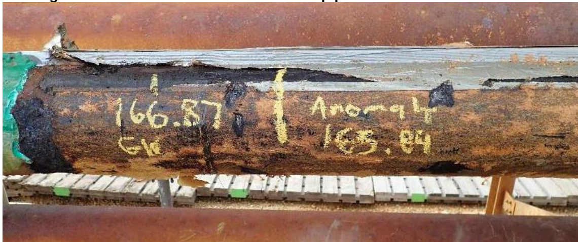
Figure 4. Section of an insulated heated pipeline after insulation removal
