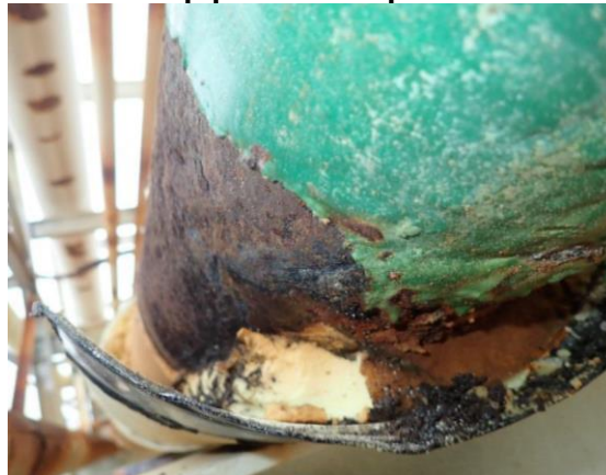
Figure 3. Insulated heated pipeline with part of the insulation removed
